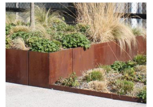
Weathering Steel, The High Line
