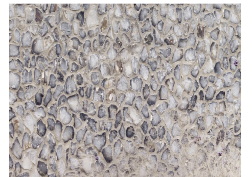
Flint Wall, Cassion Castle Architects
